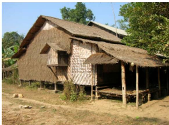
(C) Partition and roofing by Thatch-panels
