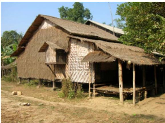
(C) Partition and roofing by Thatch-panels
